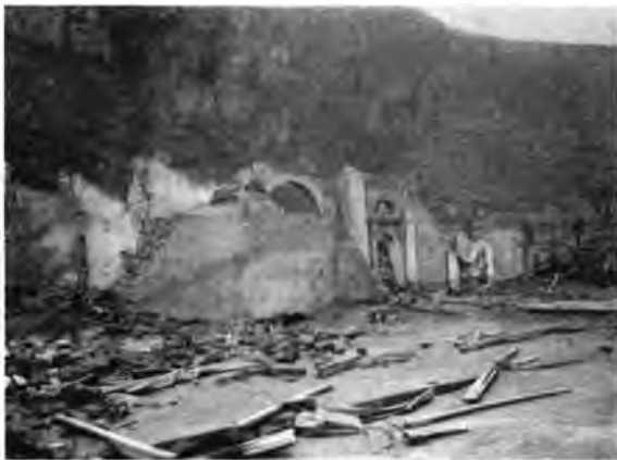
REMAINS OF A FINE PRIVATE HOUSE NEAR THE BLUFF , ST. PIERRE
